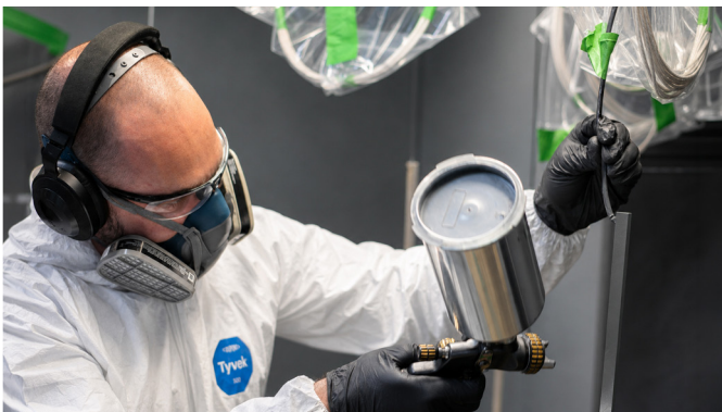
Application of a semi-conductive coating
